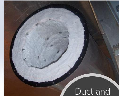
Duct and plenum are internally insulated
