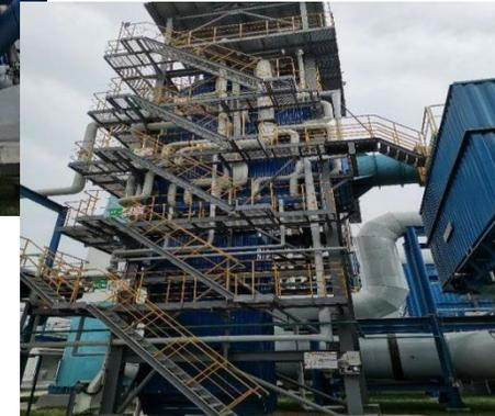
Heating and power generation system adopting RTO technology for ultra-low concentration coal mine gas(1% to 1.2%).
