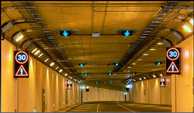
Typical VMS are using different ways for light emitting and reflecting, e.g. LED technology or rotating prisms, used in side tunnels, in hot and cold environment
