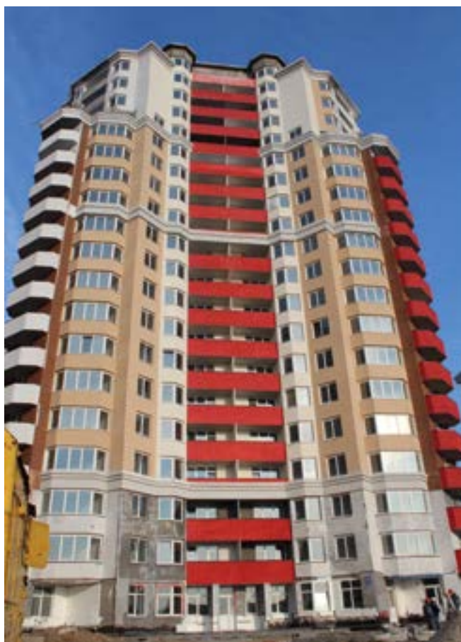
Picture 5. A social housing under construction
