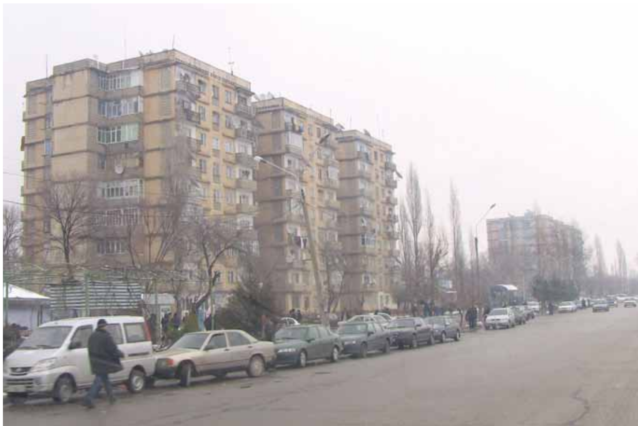
Picture 8. Multifamily housing in need of upgrading
