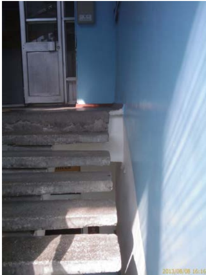
Picture 6. A staircase in one of the public offices in Chisinau
