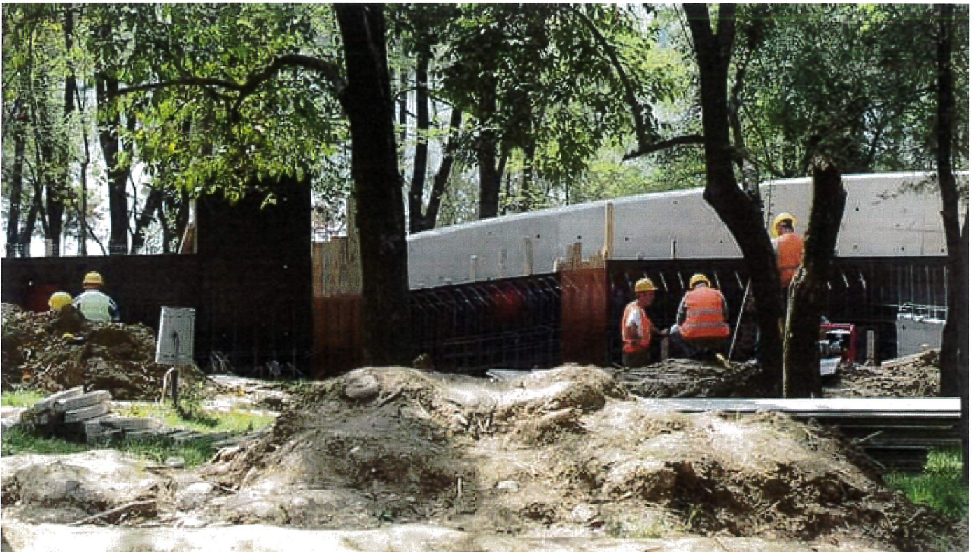
Construction work on the “children’s playground” in the Lake Park
