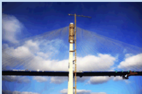
Photography: BongEui Hong, Incheon Bridge Co.,Ltd.
