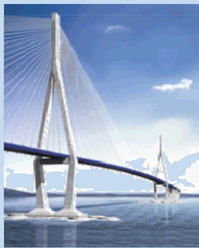
Photography: BongEui Hong, Incheon Bridge Co.,Ltd.
