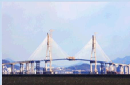
Photography: BongEui Hong, Incheon Bridge Co.,Ltd
