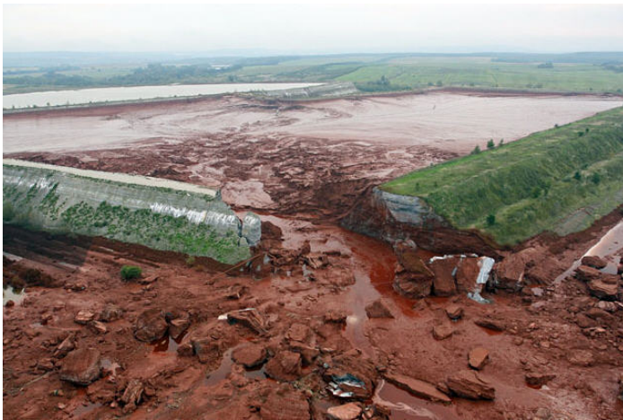
Red Sludge Spill, 2010
