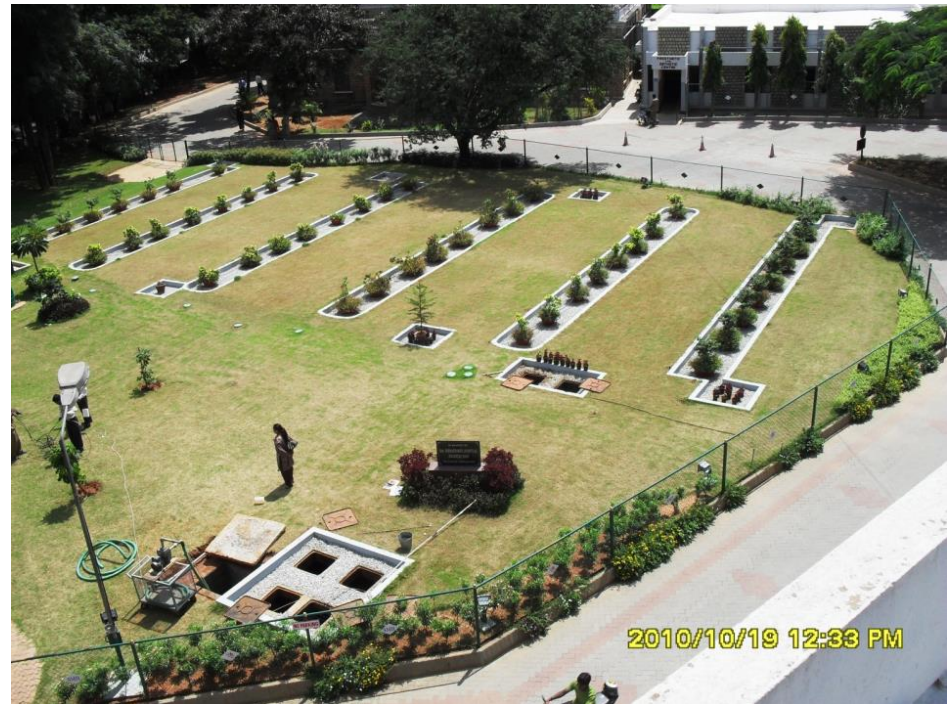
DEWATS in Bangalore
