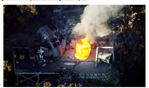
Figure 2. Fire at the upcast shaft following the third explosion
