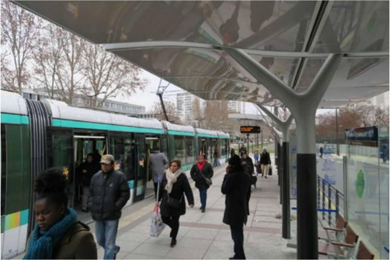
FIGURE 3.15 PARIS. ALL THE TRAMWAY STOPS ARE EQUIPPED WITH PLATFORMS, LEVEL WITH THE VEHICLE FLOOR, ALLOWING NOT ONLY CONVENIENT ACCESS FOR EVERYBODY, BUT ALSO REDUCING BOARDING TIME. EVERY PLATFORM HAS A SPECIAL WAITING AREA WITH ENOUGH WIDTH AND SEATS. THE TYPICAL STOP IS EQUIPPED WITH AN INFORMATIONAL TABLE ON WAITING TIME FOR THE ROUTES SERVED
