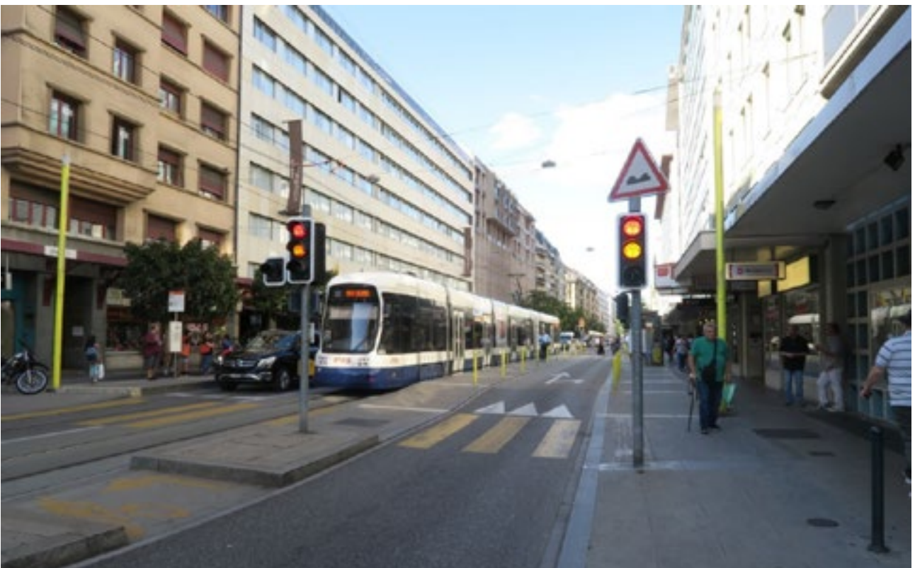
FIGURE 3.46 GENEVA. THE ROAD PAVEMENT IS RAISED AT STOP AREA TO THE PLATFORM LEVEL, PROVIDING NOT ONLY CONVENIENT BOARDING FOR THE PASSENGERS, BUT ALSO SAFETY ON BOARDING AND PRIORITY FOR TRAM MOVEMENT. THIS TYPE OF TRAM PLATFORM IS CALLED “WIEN PLATFORM”
