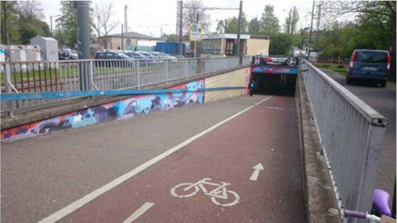
FIGURE 3.9 DÜSSELDORF, GERMANY. RAMP FOR GRADE-SEPARATED CROSSING OF BIKE LANE WITH RAILROAD PROVIDES SAFE AND CONVENIENT SEAMLESS TRAVEL FOR CYCLISTS
