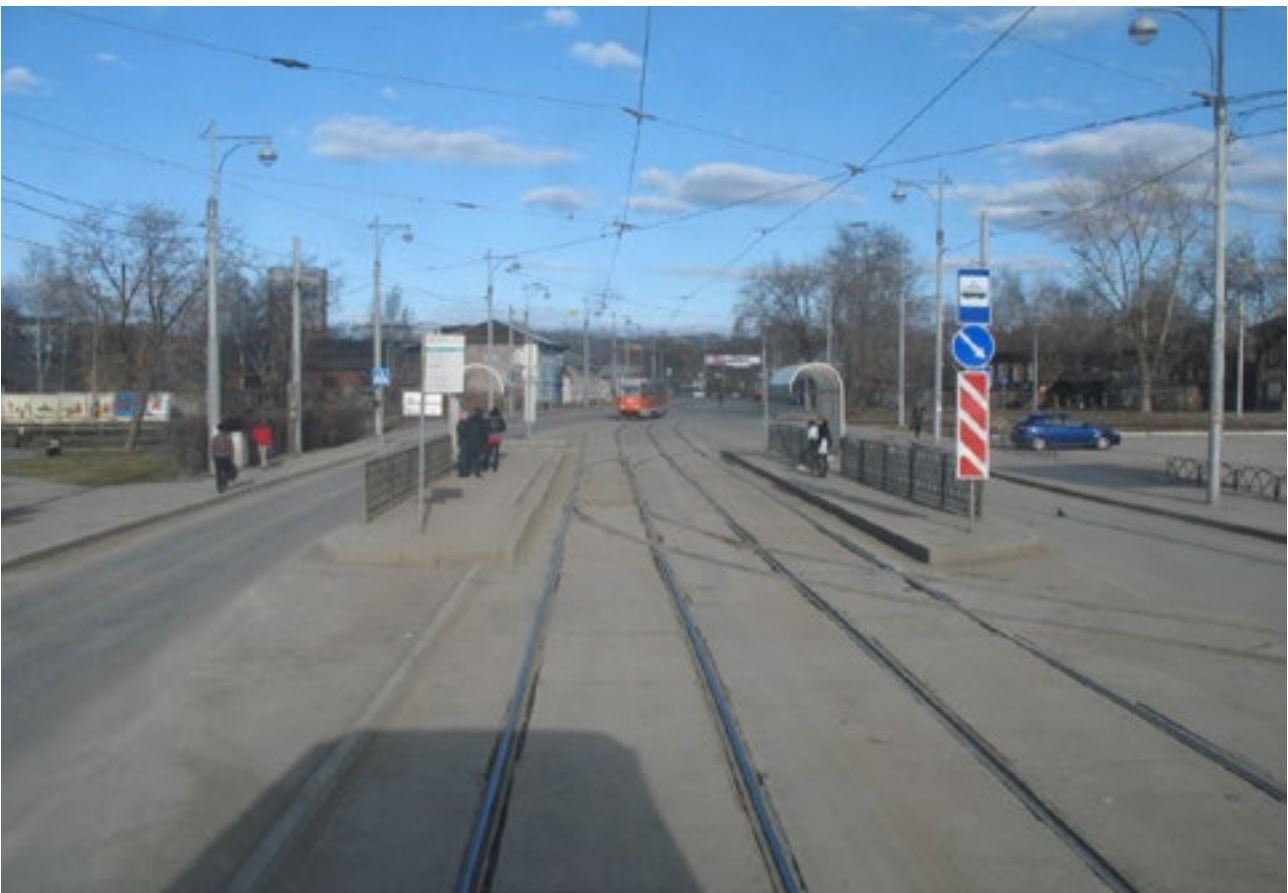
FIGURE 3.42 PERM. TRAMWAY STOP OUTSIDE OF THE CITY CENTRE IS EQUIPPED WITH ISLE PLATFORMS, PROVIDING SAFE BOARDING TO THE TRAM EVEN ON THE NARROW STREET. NOTE THE PLATFORM LEVEL ON THE EXTERNAL CURVED PART OF THE TRACK
