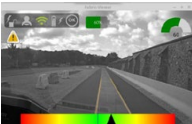
FIGURE 6.19 EXPERIMENTAL ENERGY ROAD: THE VERSAILLES-SATORY CHARGING INFRASTRUCTURE FOR DYNAMIC WIRELESS POWER TRANSFER SYSTEMS TESTING 167
