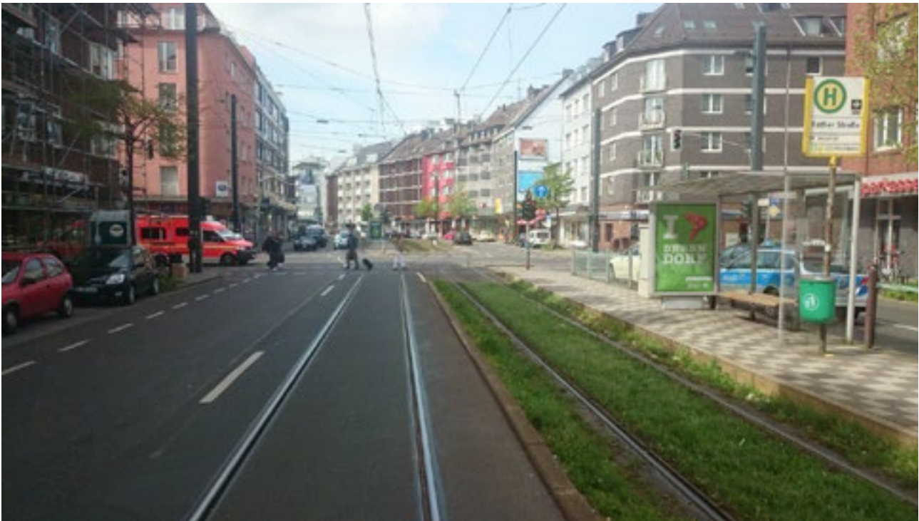
FIGURE 3.44 DÜSSELDORF. INDIVIDUAL SOLUTION TO SEPARATE ONLY ONE WAY OF TRAM TRACK IN NARROW STREET CONDITIONS
