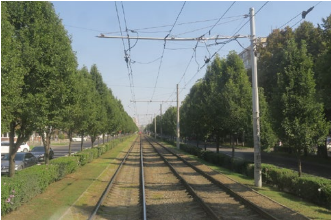
FIGURE 3.2 KRSNODAR, RUSSIAN FEDERATION. THIS LIGHT RAIL LINE DEPLOYED IN THE CENTRE OF THE AVENUE IN ORDER TO REDUCE CROSSINGS AND RAISE THE SPEED OF TRAM TRAINS. THE LINE IS SURROUNDED BY THE TREES FOR ECOLOGICAL AND AESTHETICAL REASONS. THE BUSHES PROVIDE THE GREEN FENCE FOR SAFETY AND HIGH-SPEED MOTION
