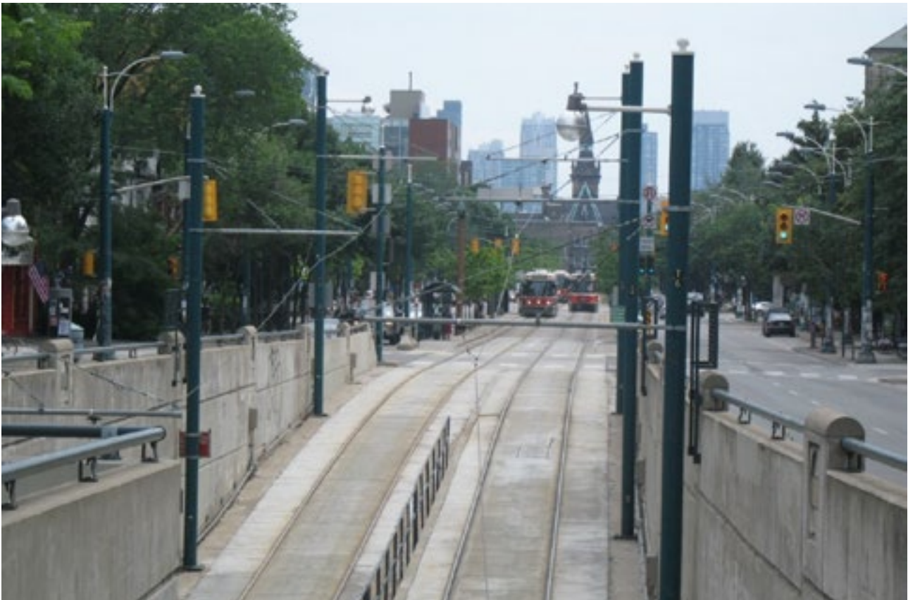
FIGURE 3.25 TORONTO. TRAMWAY LINE BUILT TO THE SUBWAY STATION BUILDING, SO AS TO PROVIDE THE SHORTEST AND MOST CONVENIENT TRANSFER TIME
