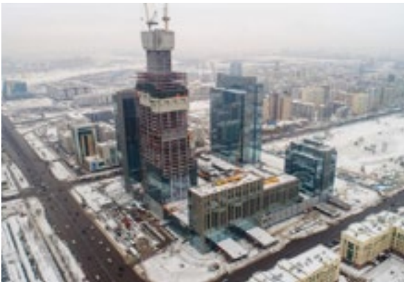
FIGURE 1.14 BU DHABI PLAZA PROJECT UNDER DEVELOPMENT IN NUR-SULTAN, KAZAKHSTAN (SOURCE: ADENMETAL)
