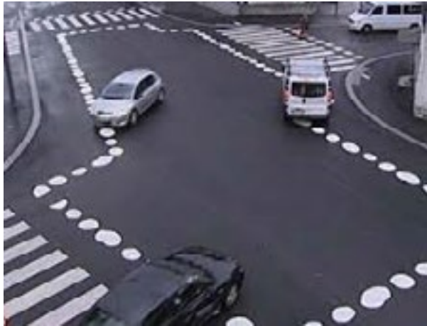
FIGURE 6.16 REDESIGNING INFRASTRUCTURES WITHOUT ELECTRONICS: THE LINDENKREUZUNG INTERSECTION IN DORNBIERN (AUSTRIA)
