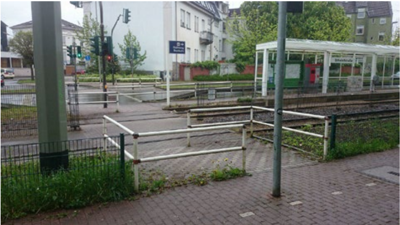
FIGURE 3.8 DÜSSELDORF, GERMANY. PEDESTRIAN CROSSING BARRIERS PROVIDES SAFE TRAM LINE CROSSING, FORCING A PEDESTRIAN TO LOOK AT COMING TRAMWAY BEFORE THE LINE CROSSING
