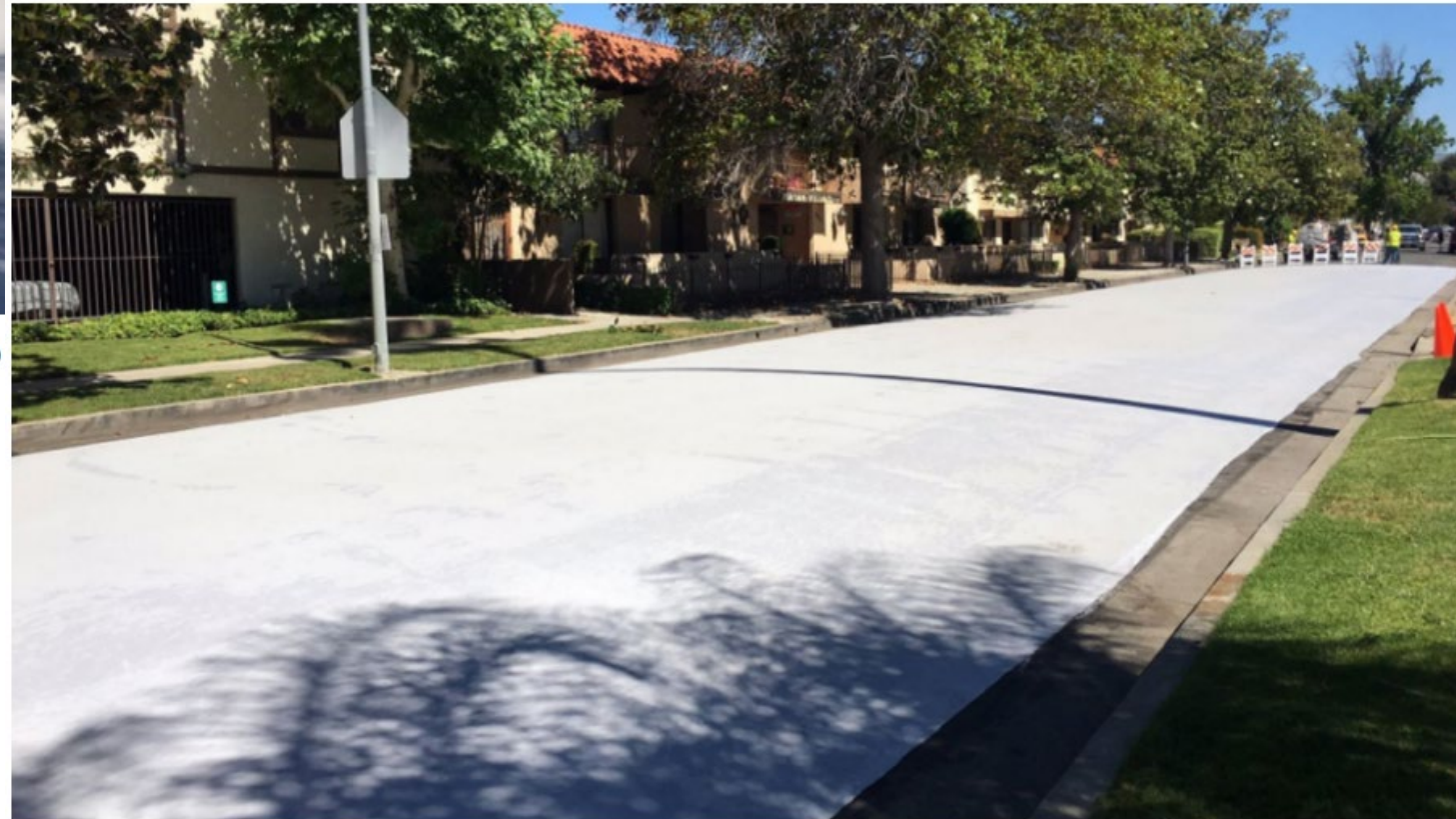
The sealant has reduced roadway temperatures by up to 10 degrees in testing. (LA Street Services)
