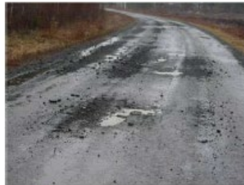
Freeze-thaw damage
