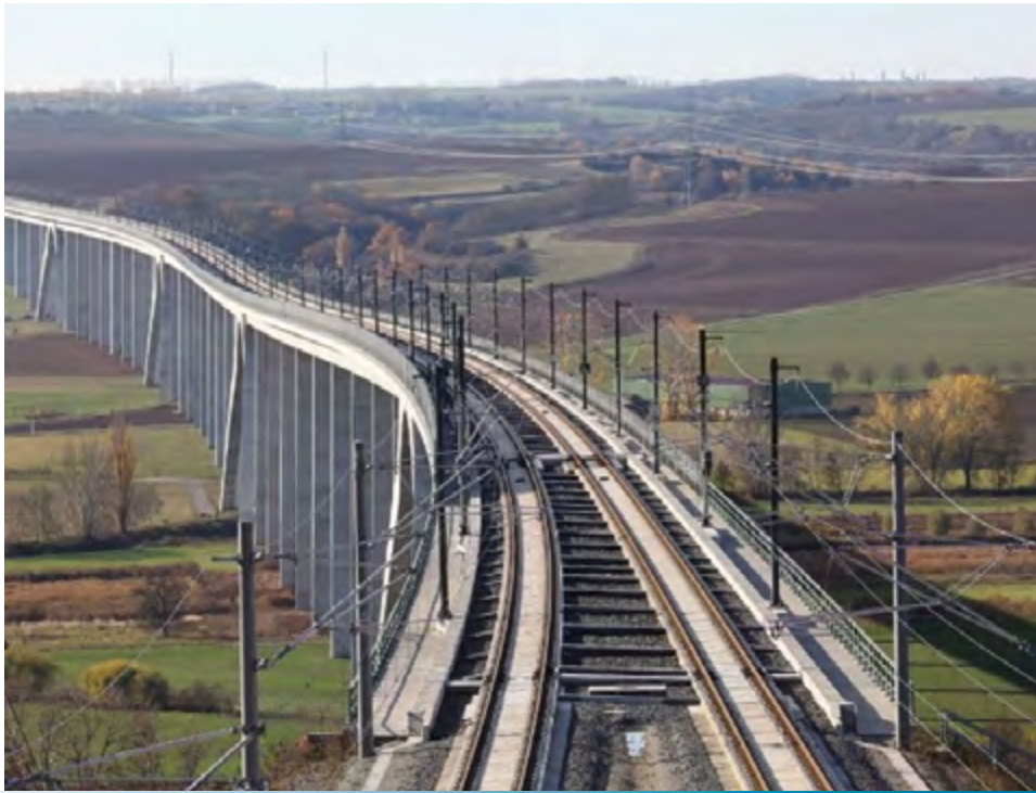
Figure 2.8 - Slab tracks on Unstrut valley bridge
