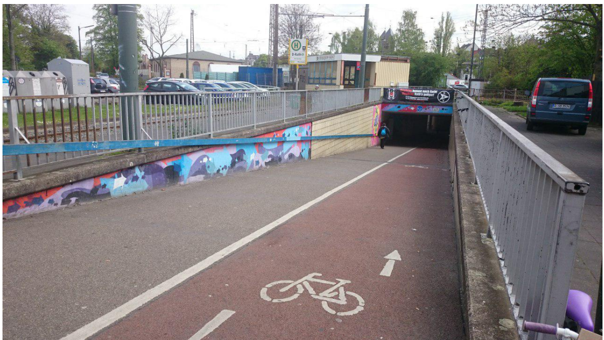
Figure 3.11. Dusseldorf, Germany. Ramp for grade-separated crossing of bike lane with railroad provides safe and convenient seamless travel for cyclists.
