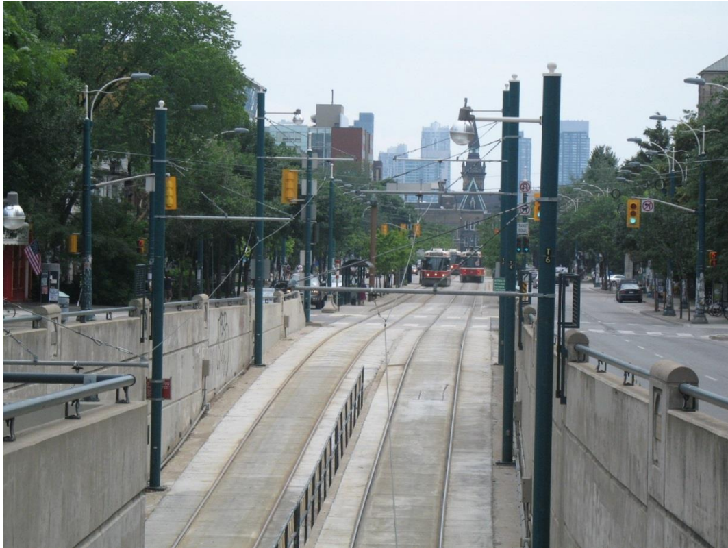
Figure 3.28. Toronto, Canada. Tramway line built to the subway station building, so as to provide the shortest and comfortable transfer.
