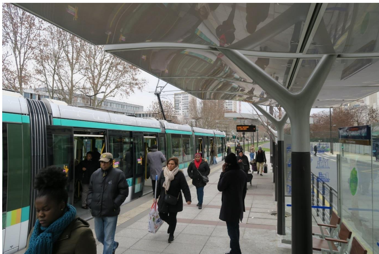
Figure 3.18. Paris, France. All the tramway stops are equipped with the platforms, levelled with the vehicle floor, allowing not only the convenient access for everybody, but also reducing the boarding time at every stop. Every platform has spacial waiting area with enough width and seats. The typical stop is equipped with informational table, providing information on waiting time for routes served
