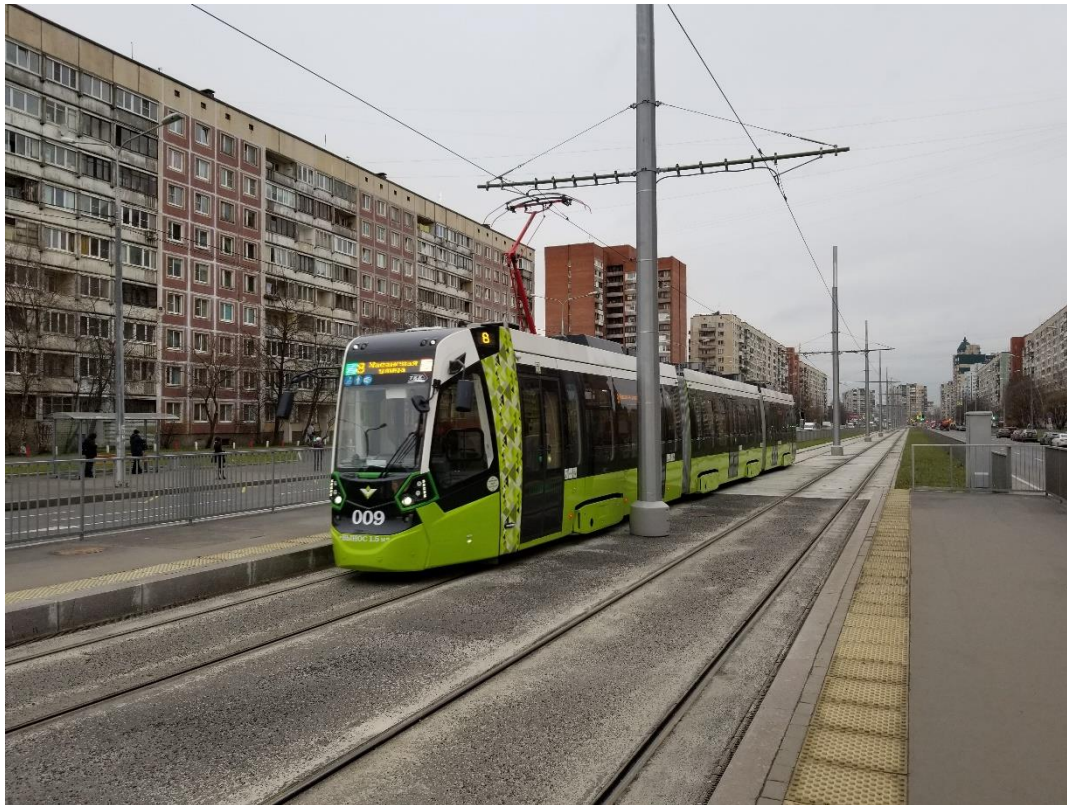
Figure 3.65. St Petersburg, Russia. The public-private partnership allows to rebuild tramway line in Krasnogvardeisky district according to the light rail standards
