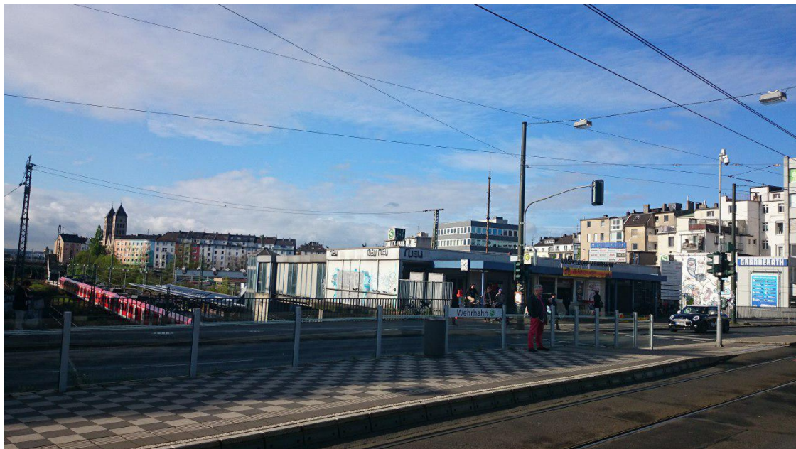
Figure 3.30. Dusseldorf, Germany. Tramway stop is placed on the railway bridge in order to minimize walking distance at transfer.
