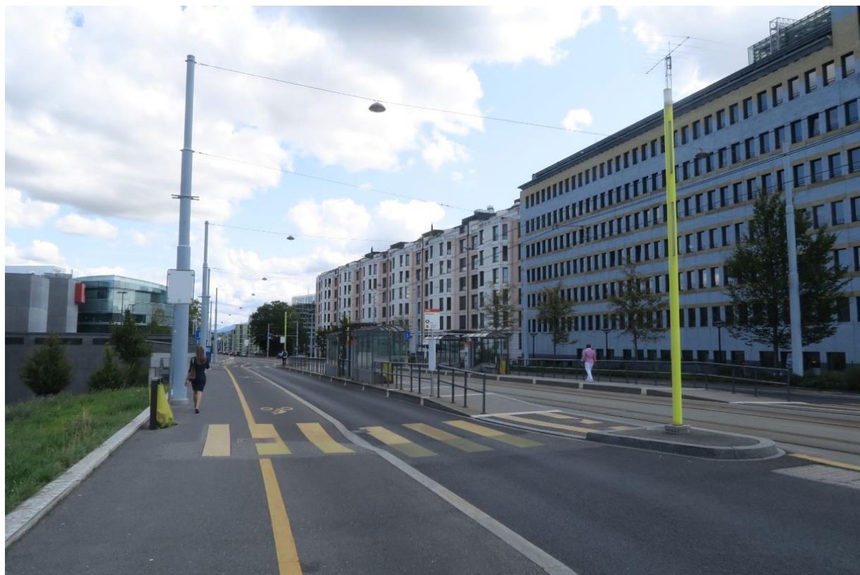
Figure 3.6. Geneva, Switzerland. The road space is divided between all the modes – rail transit, pedestrians, bikes and cars. Only single line is provided for cars.
