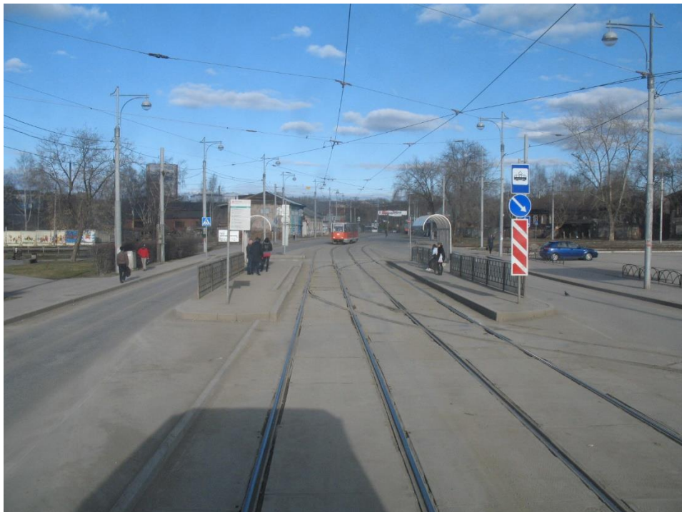
Figure 3.55. Perm, Russia. Tramway stop outside of the city center is equipped with isle platforms, providing safe boarding to the tram even on the narrow street. Note the platform level on the external curved part of the track.
