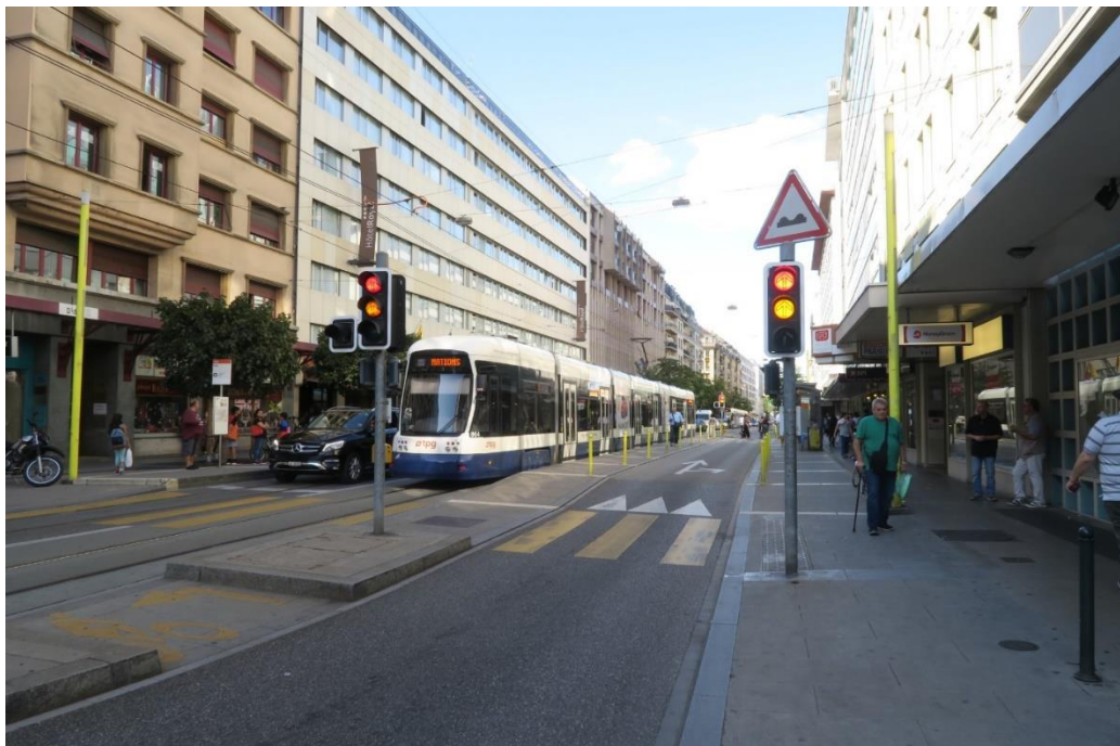
Figure 3.59. Geneva, Switzerland. The road pavement is risen at stop area to the platform level, providing not only convenient boarding for the passengers, but also the safety on boarding and priority for tram movement. This type of the tram platform is called “Wien platform”.
