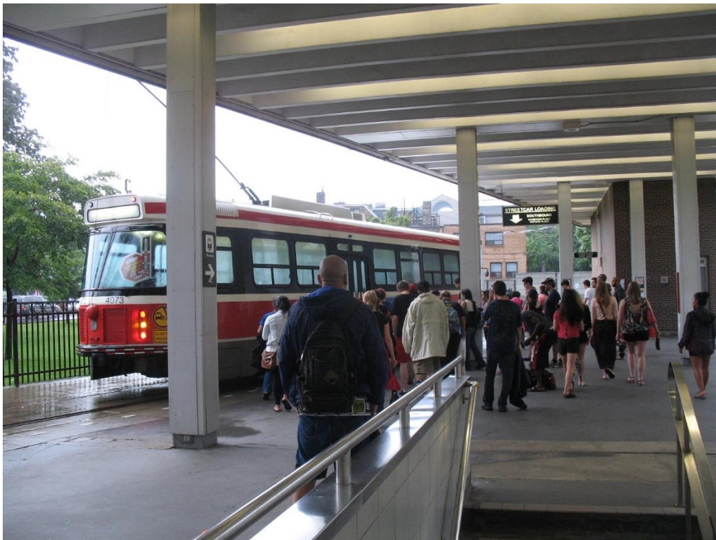
Figure 3.28. Toronto, Canada. Tramway line built to the subway station building, so as to provide the shortest and comfortable transfer.
