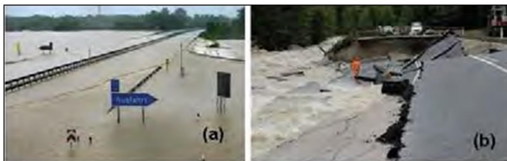
Figure 12 Flood damages on European roads in June 2013: (a) Highway 8 in Grabenstaett, S. Germany ((Matthias Schrader, AP); (b) Tyrol, Austria ( Kerstin Joensson, AP).
