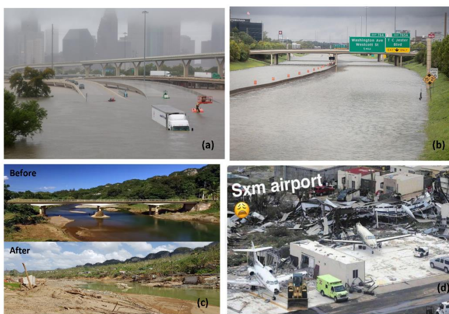
Figure 14 Transport infrastructure damages from the 2017 hurricanes. (a) Harvey: highway flooding in downtown Houston (USA) ( https://www.pbs.org/newshour/science/hurricane-harvey-became-extreme ). (b) Harvey: Houston highways ( https://www.vox.com/science-and-health/2017/8/28/16211392/100-500-year-flood-meaning ). (c) Maria: Bridge at Puerto Rico ( https://coastalresiliencecenter.unc.edu/2018/10/lessons-learned-from-hurricanes-irma-and-maria/ ). (d) Destruction of the Sintt Maarten Princess Juliana international airport by Hurricane Irma (September 2017) ( https://sxmgovernment.com/2017/09/07/new-photos-hurricane-irmas-destruction-of-st-maartens-princess-juliana-international-airport/ )
