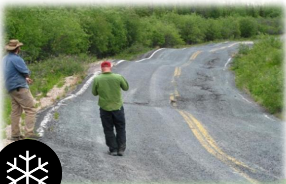
Permafrost degradation, Dempster Highway, NWT
