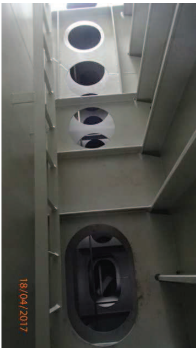
Water Ballast tank no 3, Portside (Webframes)
