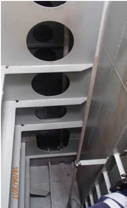
Water Ballast tank no 1, Portside (Web frame)
