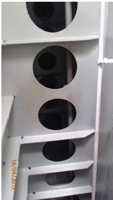
Water Ballast tank no 2, Portside (Web frame)
