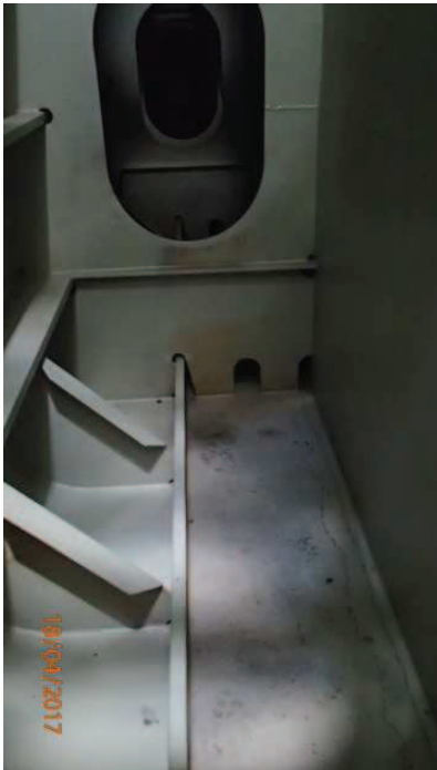
Water Ballast tank no 1, Portside (Bottom plating)
