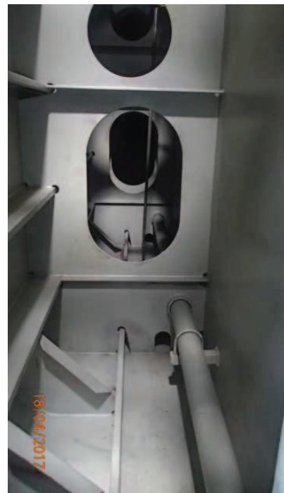
Water Ballast tank no 2, Portside (Bottom plating)
