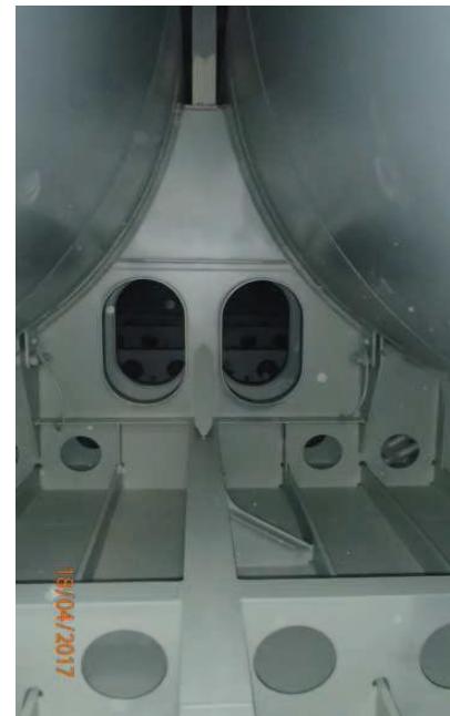
Aft void space (Cargo tank Foundation)
