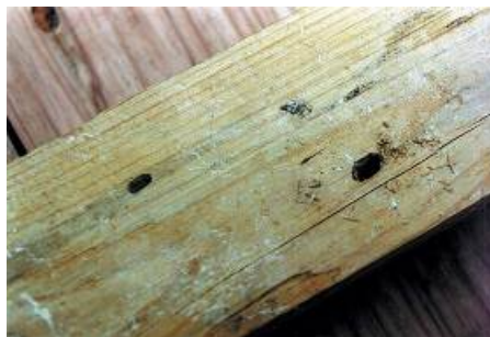
Figure 6.13 Wood frass from boring insect
