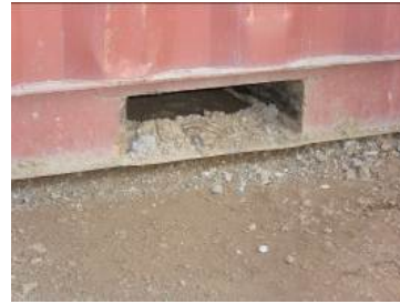
Figure 6.3 Mud in fork pocket
