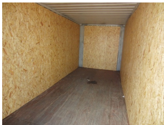
Figure 7.53 Lining a 40-foot container with chipboard panels
