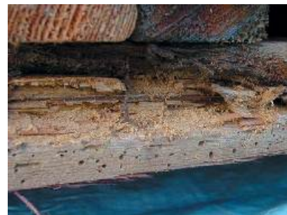
Figure 6.13 Wood frass from boring insect
