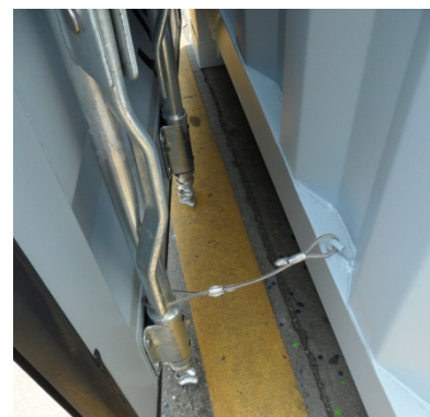
Figure 5.30 Door retaining strap
