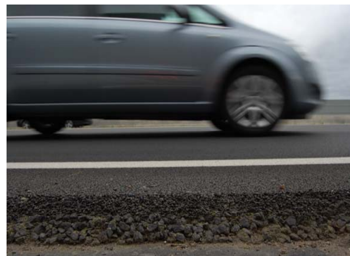
figure 1: double layered asphalt
