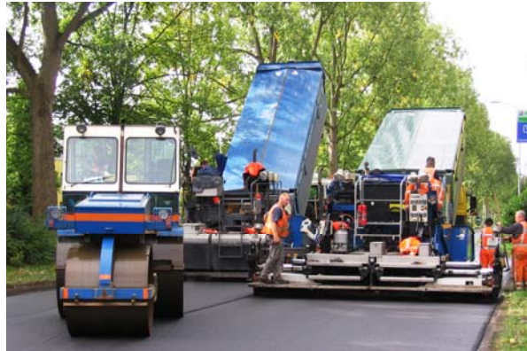
Figure 5: laying quiet road surface
