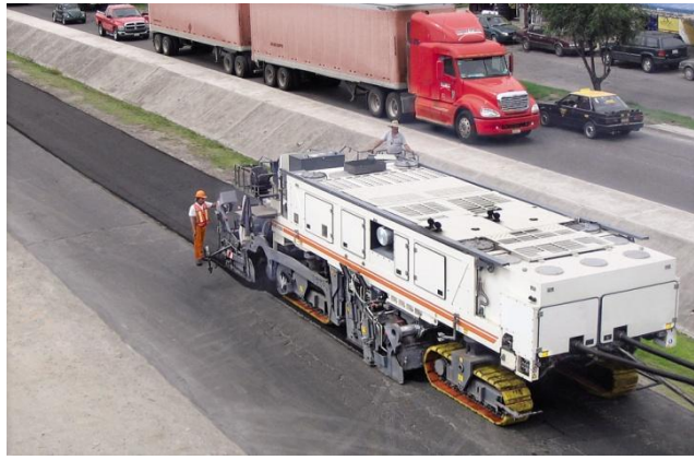
Cold recycler in operation
