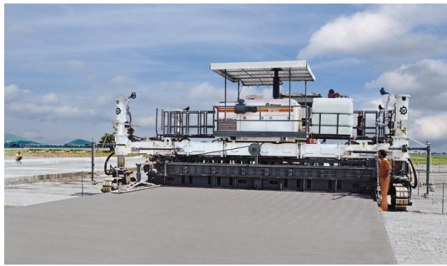
Slipform paver in operation
