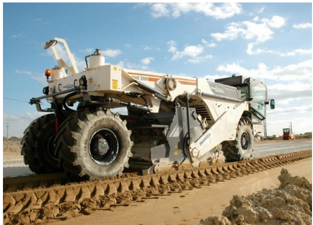
Cold recycler/soil stabilizer in operation
