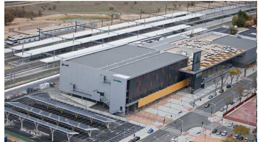
PHOTOVOLTAIC PANELS ON THE PARKING OF THE ALBACETE STATION (Source ADIF 2010)
