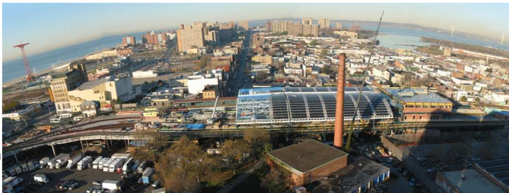
SOLAR PANELS ON THE ROOF OF STILLWELL AVENUE STATION (Source NYCT 2004)
