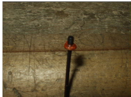
Figure 131 - Add Sealant to Cover Screw
