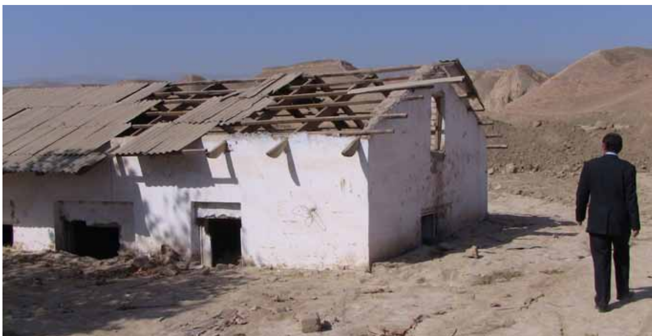
Picture 1. Family house destroyed by a landslide, Vanj district
