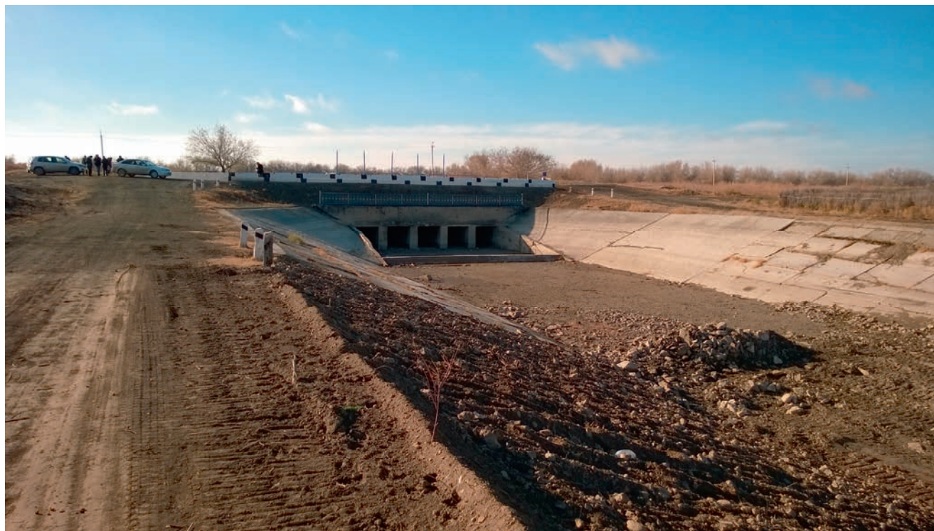
Photo 11.6: Muynak Canal Head at Mezhdurechensk Reservoir
