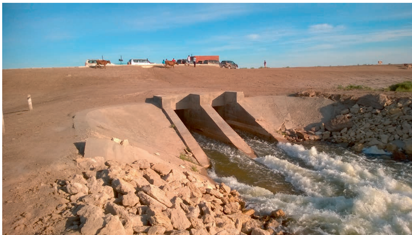
Photo 11.5: Water outlet, Rybachye Reservoir
