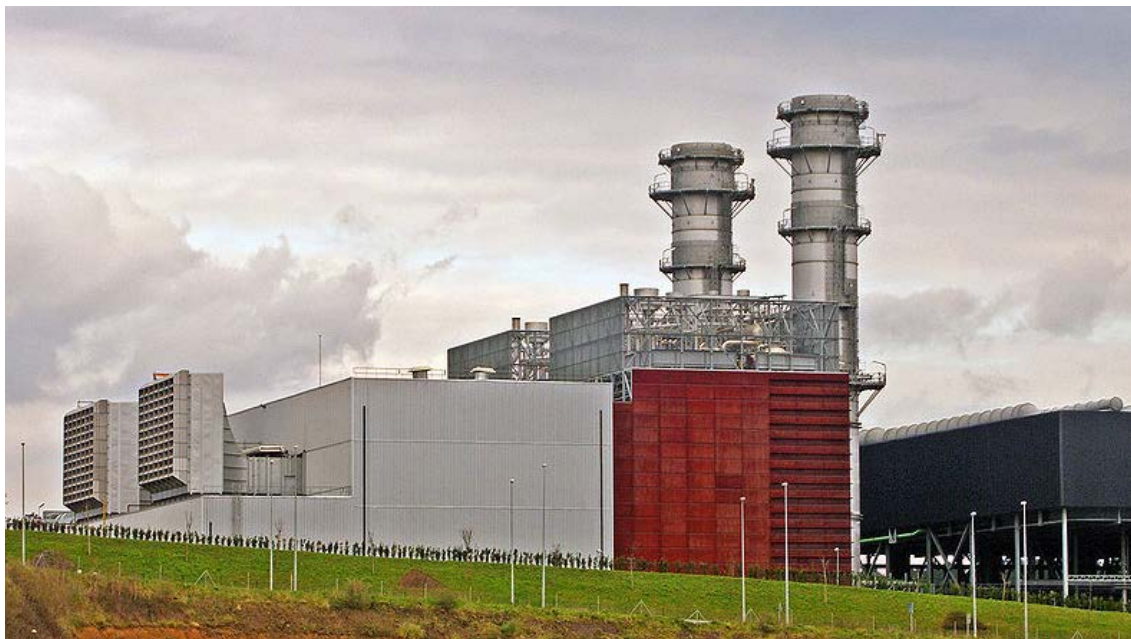
Figure 35 – Photo of a Combined-Cycle Gas Turbine (CCGT) Plant
