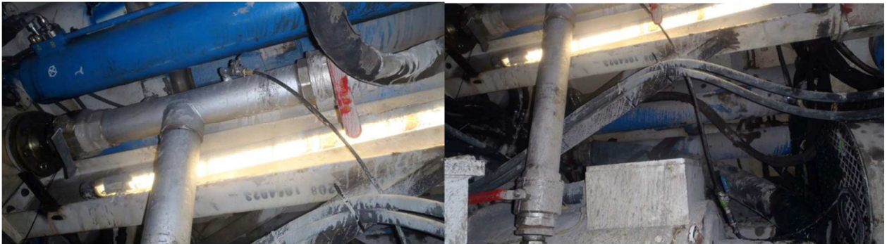
Figure 11: Methane sampling/bleed hose (left) behind the cutter bulkhead (right).
