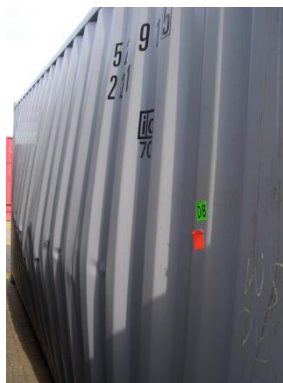
Figure 7.70 Bulging wall
