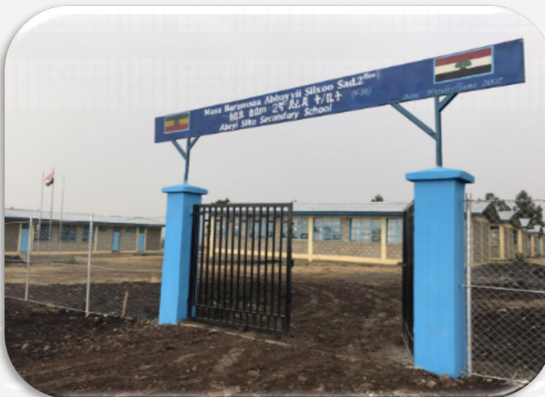
GEIDCO's Assistance to the Abay Silto School Power Supply Project in Ethiopia
