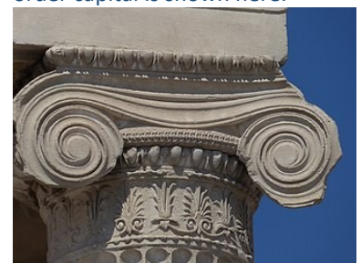
C. The Ionic order is one of the three canonic orders of classical architecture, the other two being the Doric and the Corinthian. The Ionic order capital is shown here.
