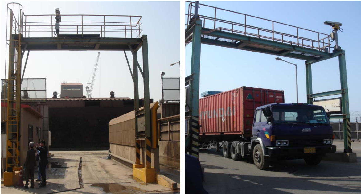
Figure B.5. Photographs of Korean Portal Monitoring System.
