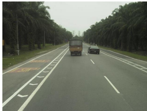
T2: Presence of auxiliary lane for acceleration on the motorcycle lane
