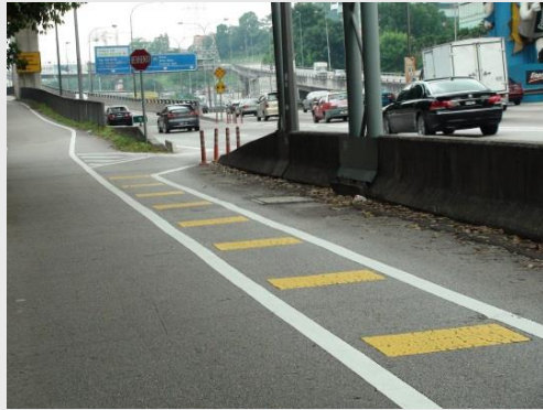
T2: Presence of auxiliary lane for acceleration on the motorcycle lane
