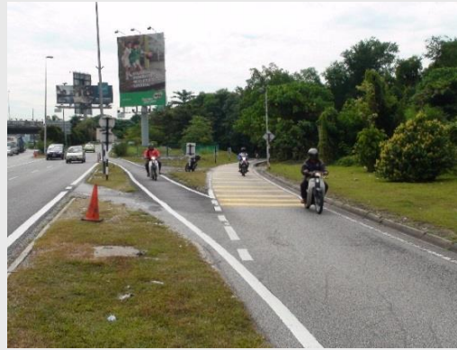
T4: Entry angle <90 degree, length of slip lane >15m
