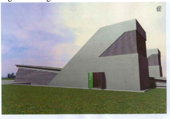
Fig. 9. Building on top emergency shaft at surface level
