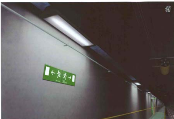
Fig 3. Lightened escape route with pictograms
