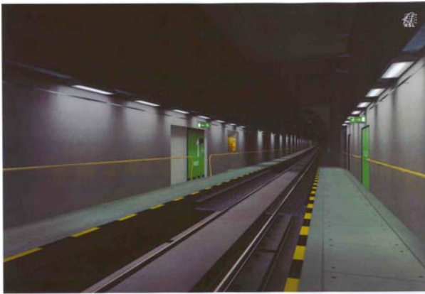
Fig. 5. Passage to emergency shafts with foot-boards to cross the track
