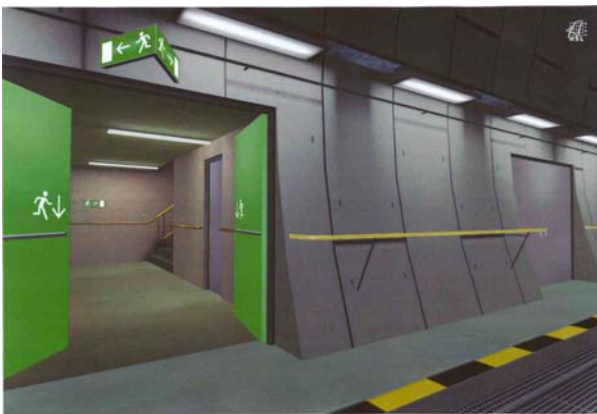
Fig. 6. Doors to emergency shafts
