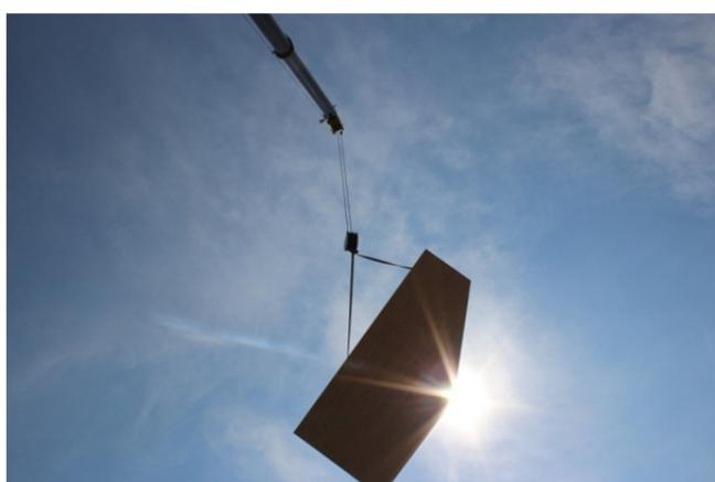
**Note:** CNC-machined CLT board being lifted to its position.
