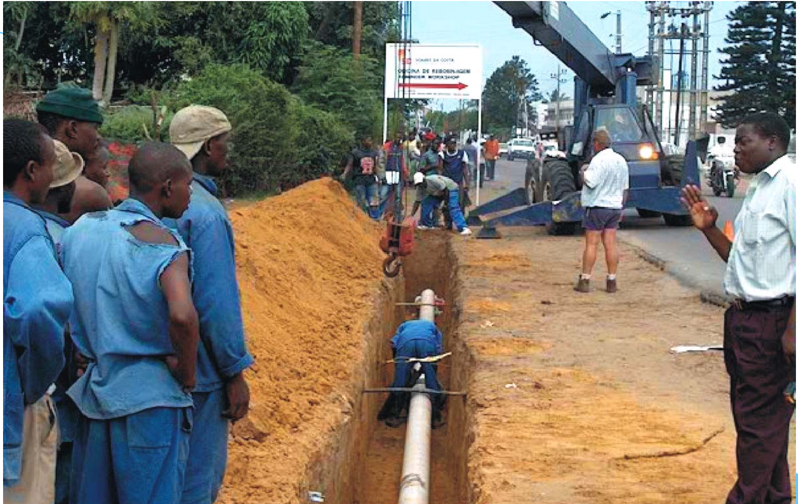
PIPELINE CONSTRUCTION IN MATOLA
