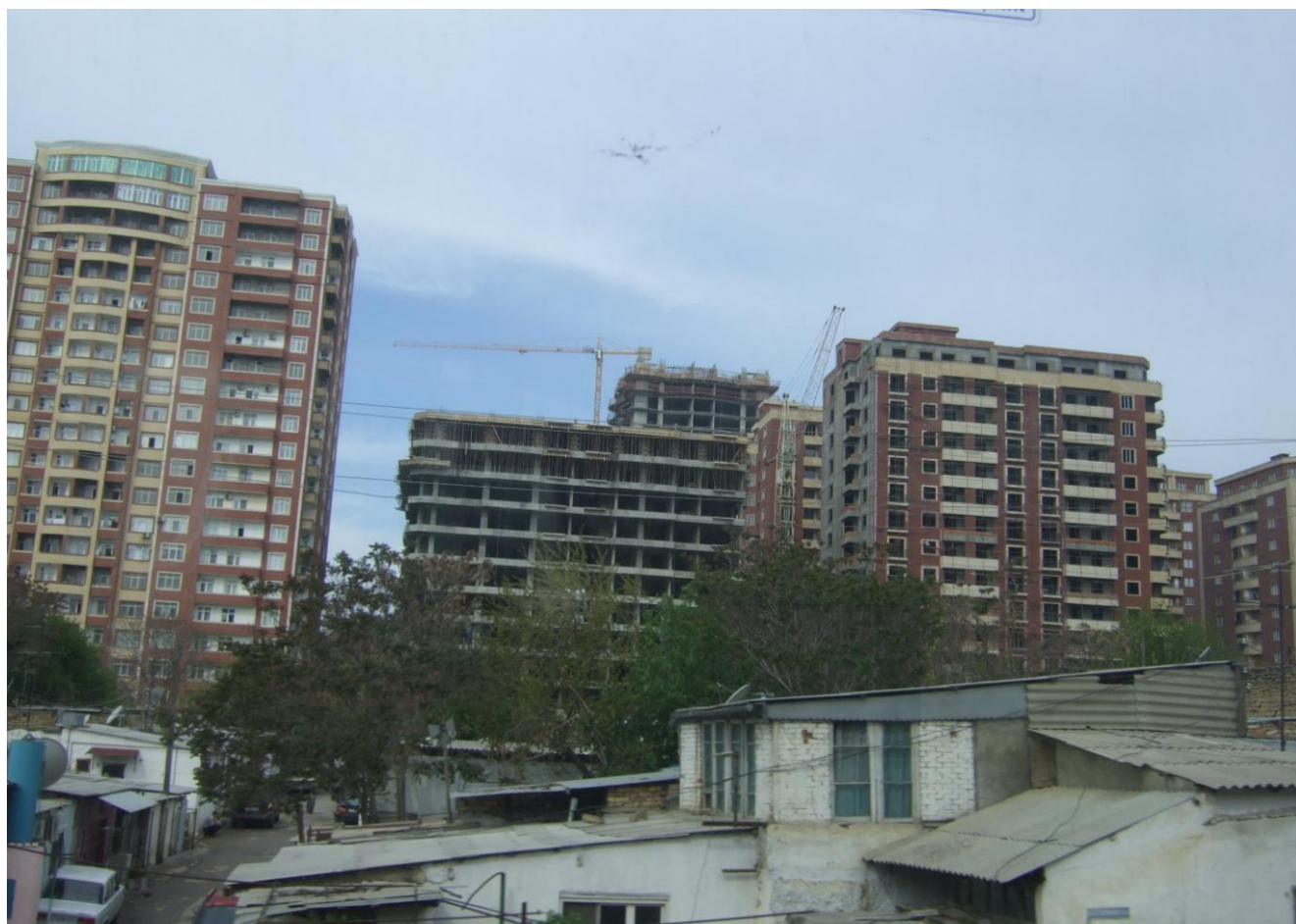
Picture 3. Multifamily housing in Baku Source: UNECE
