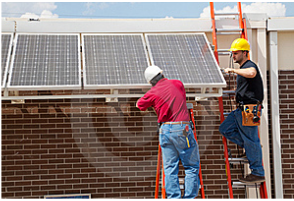
Men installing solar panels in Eastern Europe (photo Lisa F. Young).
