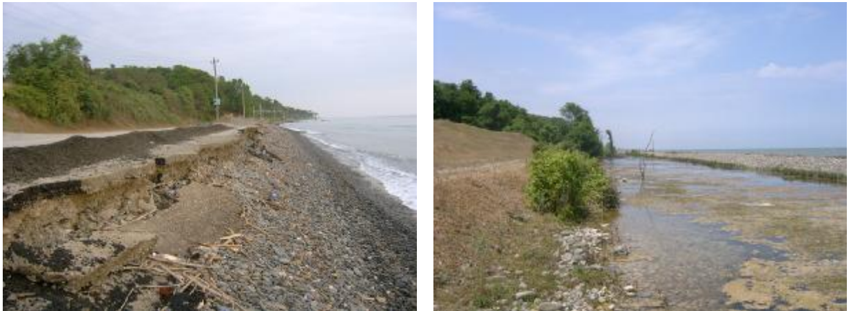
Fig. 7. Examples of flooding coastal zone in result rising Caspian Sea level.
