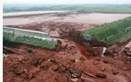
The TMF at Ajka (Hungary) after the dam failure (2010)
