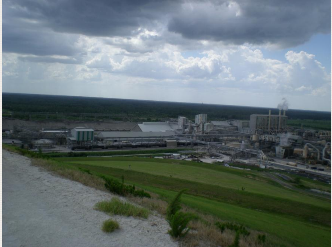
Uranium extraction plant at a phosphate fertiliser plant, Florida USA (not in current use)
