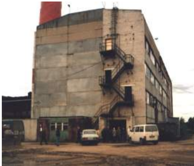
Central Heating Station Kaljasin
