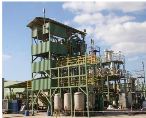
Lab Scale 150 kWth CFB Gasifier
