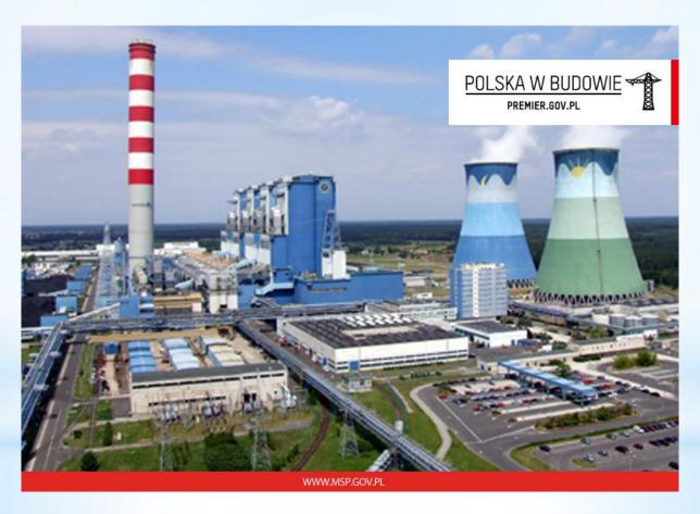
OPOLE P.P.  $1492 \text{ MW} + 2 \times 900 \text{ MW} \text{ (} n = 45,5\%\text{)}$
