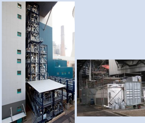
CO 2 -Scrubber since 2009 → CO 2 -Capture CO 2 -Filling station since 2011 → CO 2 -Utilisation
