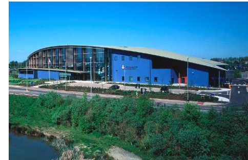
2006 Gloucester Police Building: 5%
