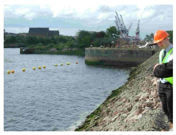
b). **Picture 2** A geotextile membrane was laid across the bund, to prevent fines from the soil being trapped in the bund or being transported into the river.
