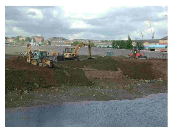
17. The area in front of the bund is to be sheet piled and a large void created, into which contaminated dredge material is to be placed and removed from the marine environment.
