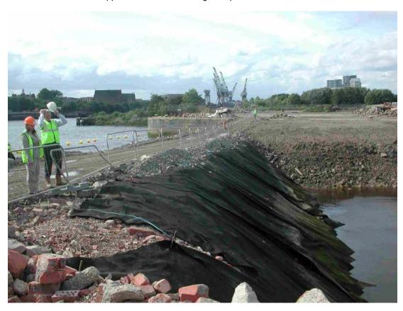
3. **Picture 3.** Tipped poor quality topsoil from within the construction site and within the planning application area (outside the material would be considered as waste, and for sale as top soil would require exemption under SEPA) is pushed by dozers into the dock and levelled.
