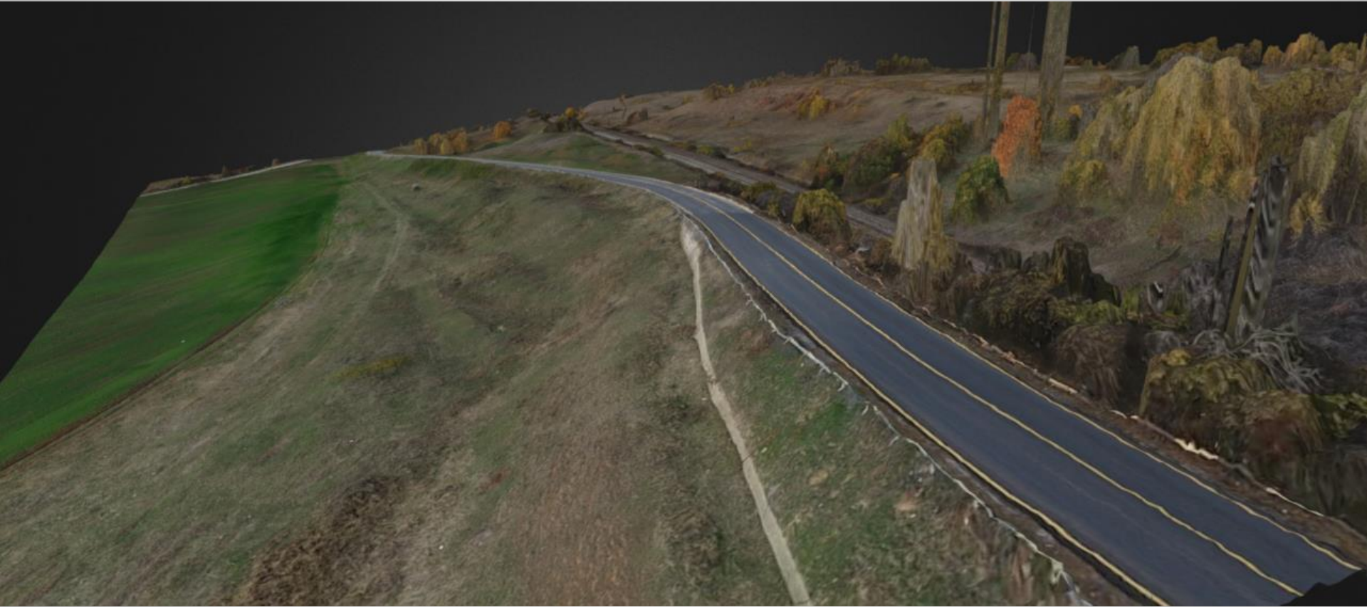
Aerial orthophoto created by project team (into problematic road sector)
