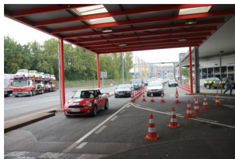
Switzerland-France Joint Border and Customs Station, Bardonnex © EuroMed RRU
