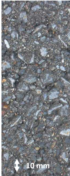
Dense asphalt concrete
